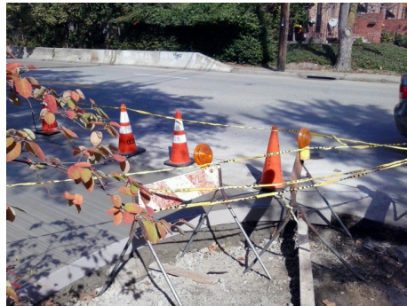
FIGURE 7.1: A wooden spline used to create a smooth, curved border for a paved area (Shadyside, Pittsburgh, October 2014).
